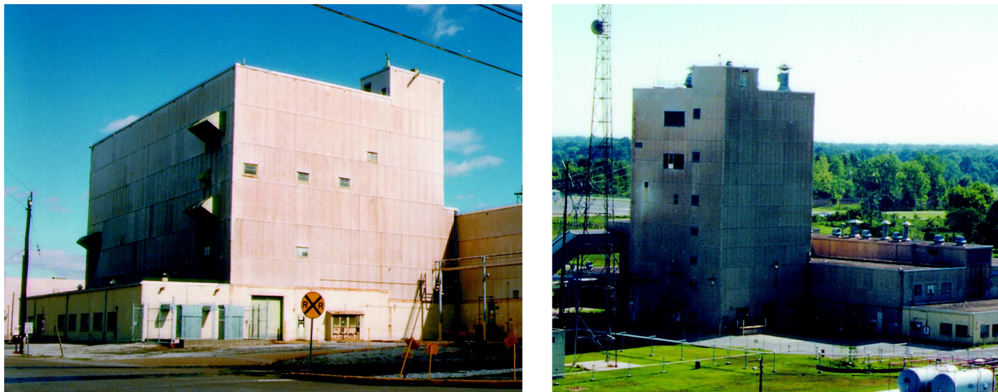
Figure 3: Two Unused, Contaminated Buildings to Be Demolished During Cleanup
